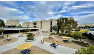
Fine Arts Building Renovation [Design - Construction Documents]
