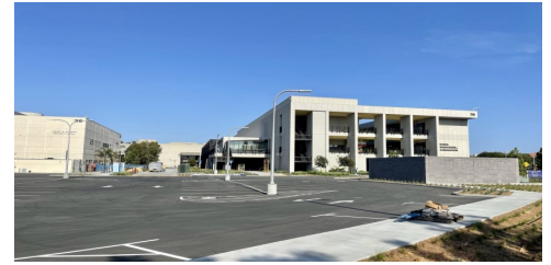
New Science, Engineering and Mathematics Building [Construction]
