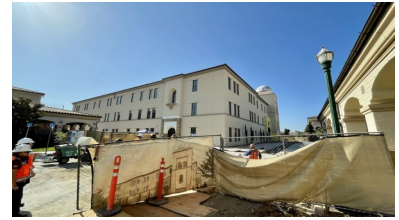
New Instructional Building [Construction]
