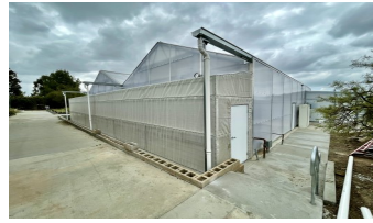
Greenhouse Replacement [Close-out]
