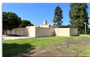
Wilshire Chiller Plant Relocation [DSA Review]
