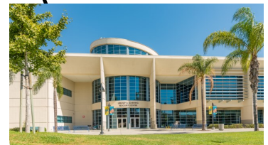
LLRC Secondary Data Center (Phase II) [Close-out]
