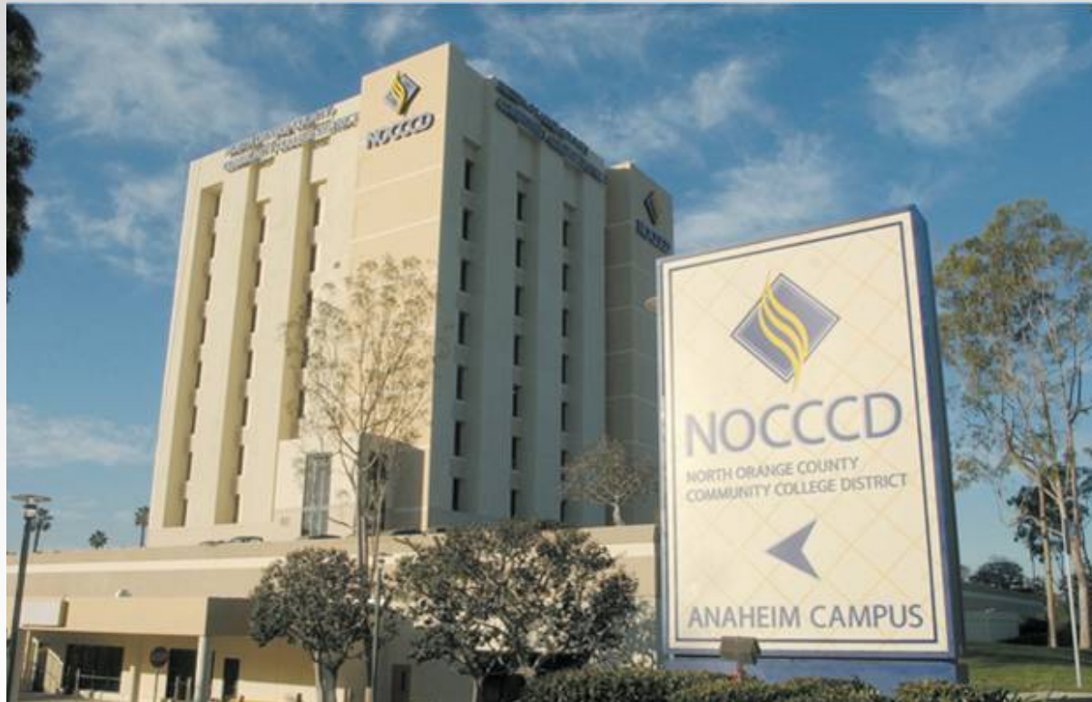
Anaheim Campus Purchase/Renovation
