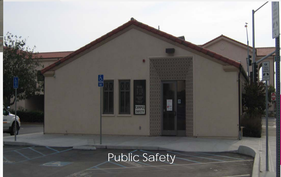
1000 Building Seismic Retrofit
