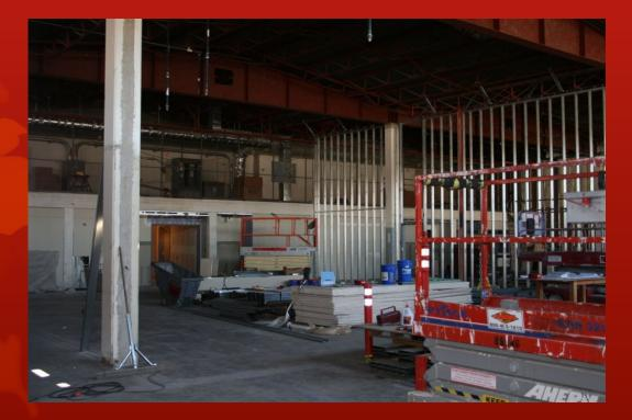
Demolition for the Welding Shop continues. Layout walls and mechanical layout exhaust duct work is also ongoing in the Welding Shop, and we are in the process of ordering materials.
