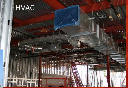
Installation of HVAC control conduits and roll-up door tube steel at South elevation has begun.
